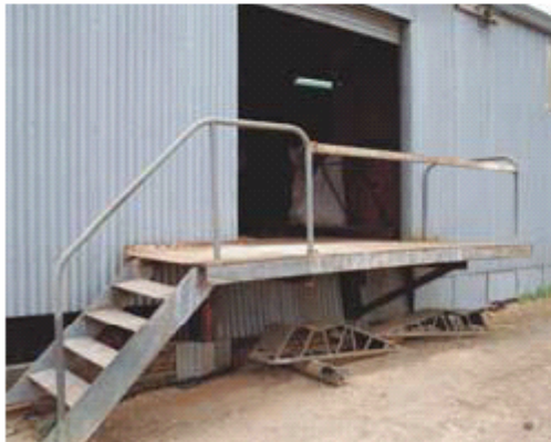
Safe access to the shed.
