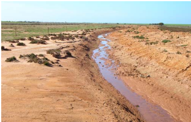
Drainage helps move surface water and groundwater across the low-lying coastal creek flats.
